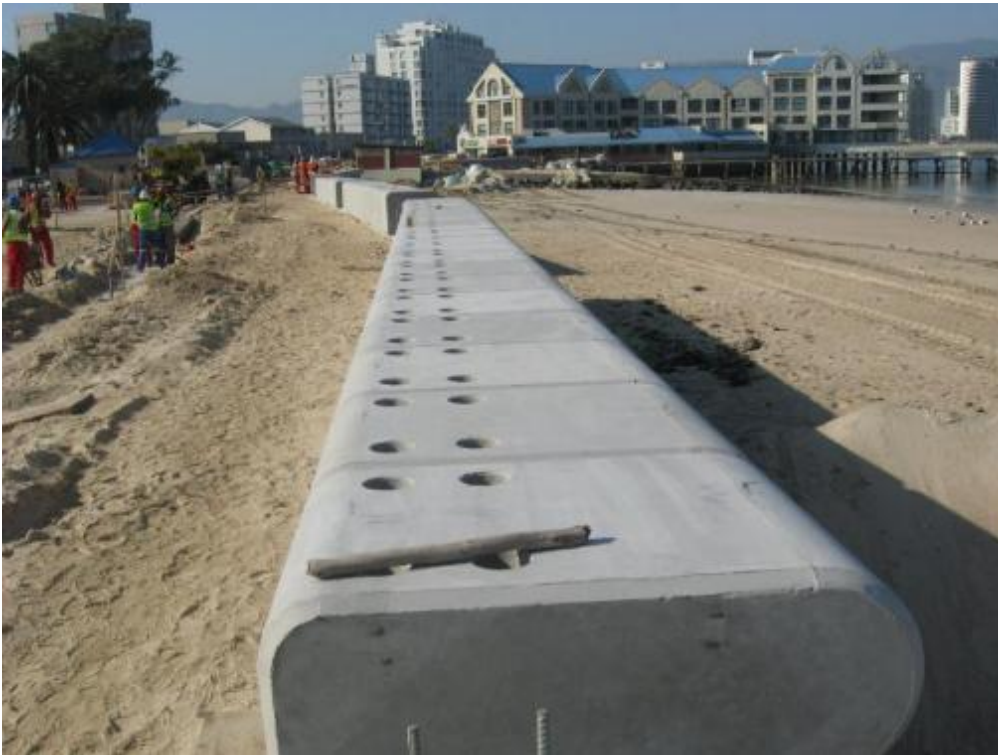
Figure 28 Seawall after backfilling. Note beach on seaward side
