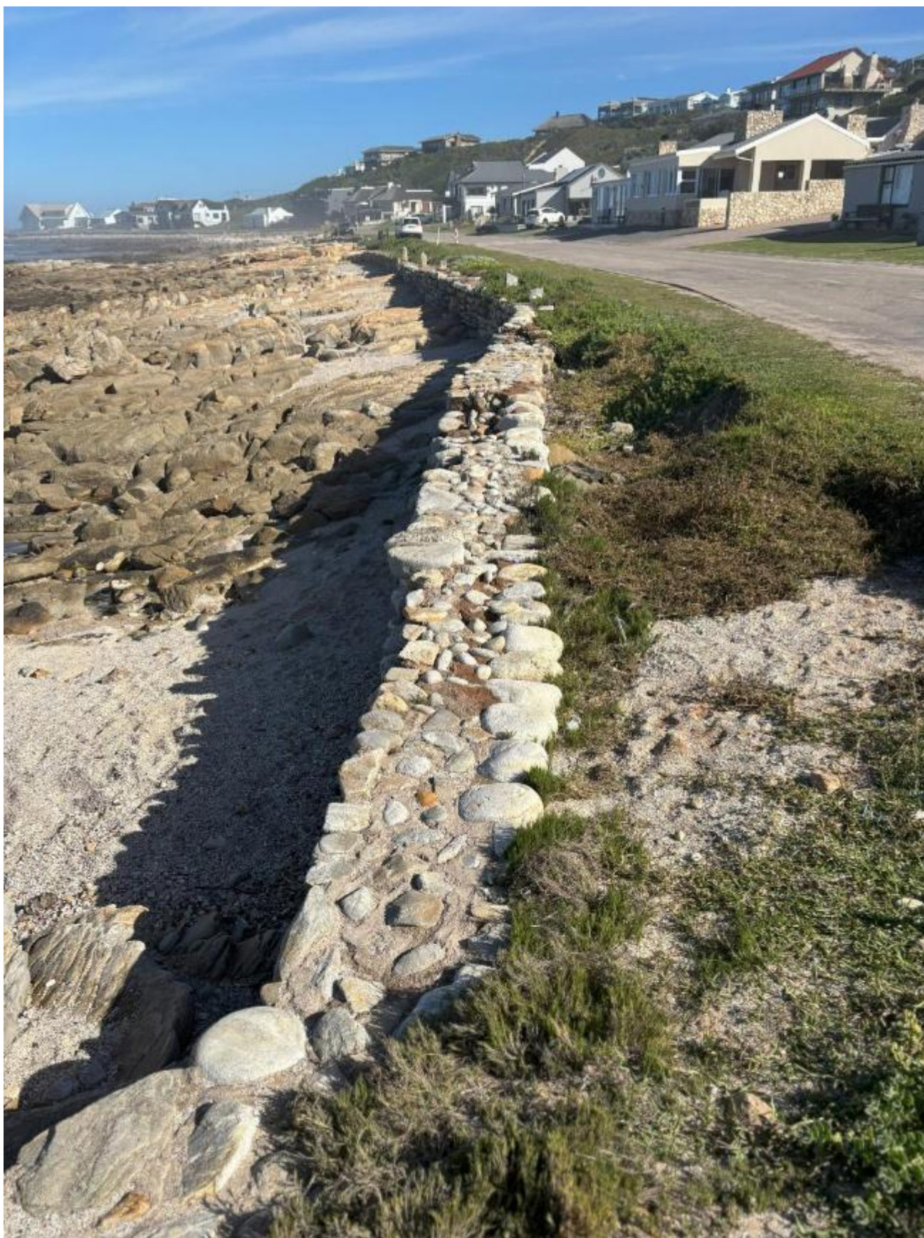
Figure 50 Natural rock masonry retaining wall from Ch320 southwards creates a 3m to 3.5m wide verge for pedestrian use – largely vegetated but showing erosion scars from storm/flood events
