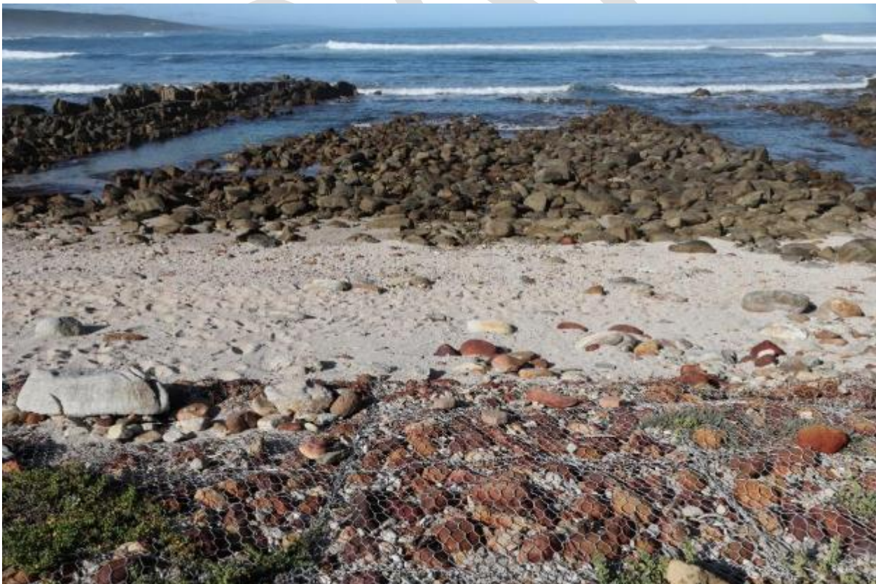
Figure 61 Seaward view Ch570 showing gabion mattress edge followed by sandy beach strip and rocky foreshore to ocean
