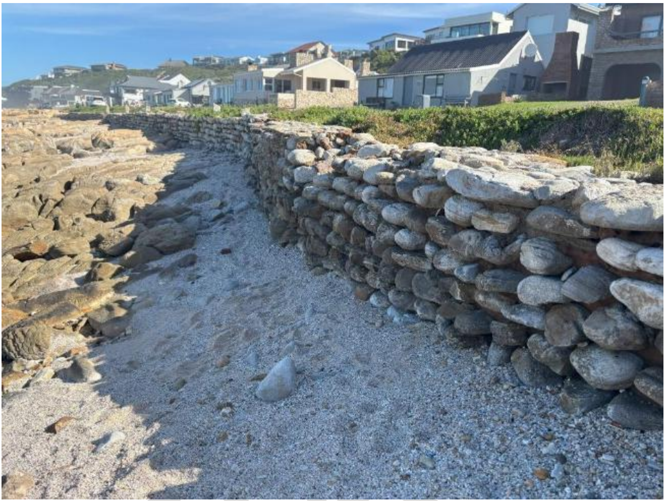
Figure 51 View from ocean side of natural rock masonry retaining wall from Ch320 southwards. Wall aesthetically pleasing and blends in with natural surroundings. Note however damage on top side from storm/flood events
