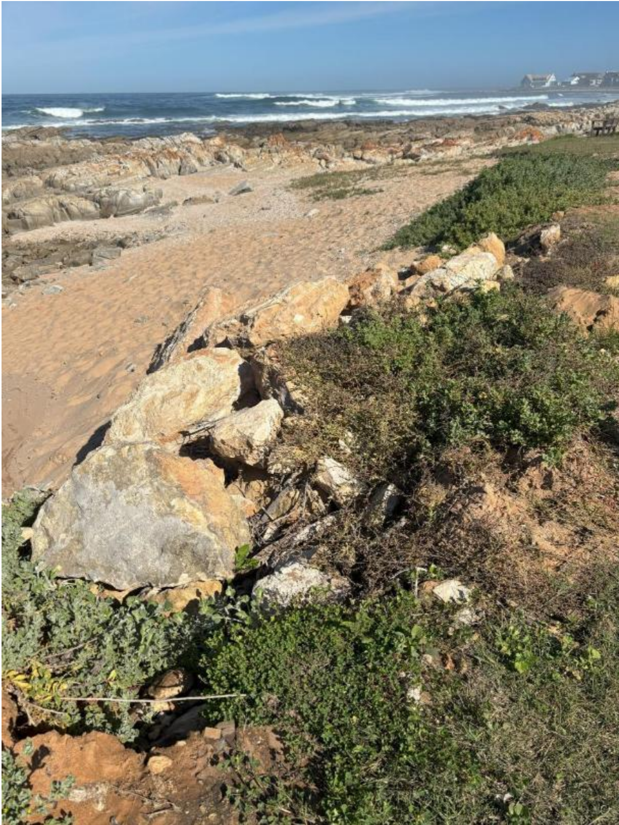
Figure 43 Ch125 looking southwards untidy and not very ineffective rock revetment supporting lawn/vegetation alongside roadway. Sound sandy upper beach area
