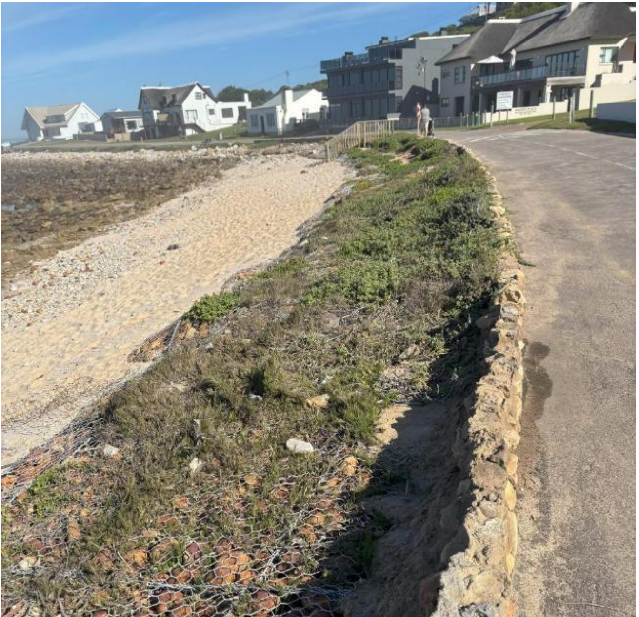
Figure 59 Gabion edging below low natural rock wall Ch550. While effective in protecting roadway these wire structures are unsightly and limit use of valuable space on the beach.
