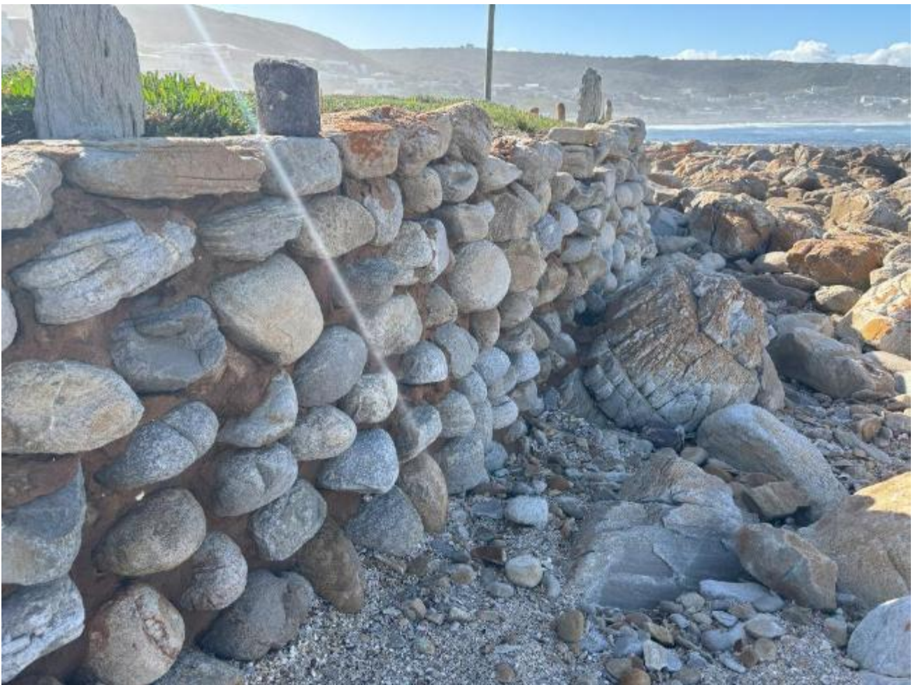
Figure 71 Natural rock retaining wall from seaward side at Ch750
