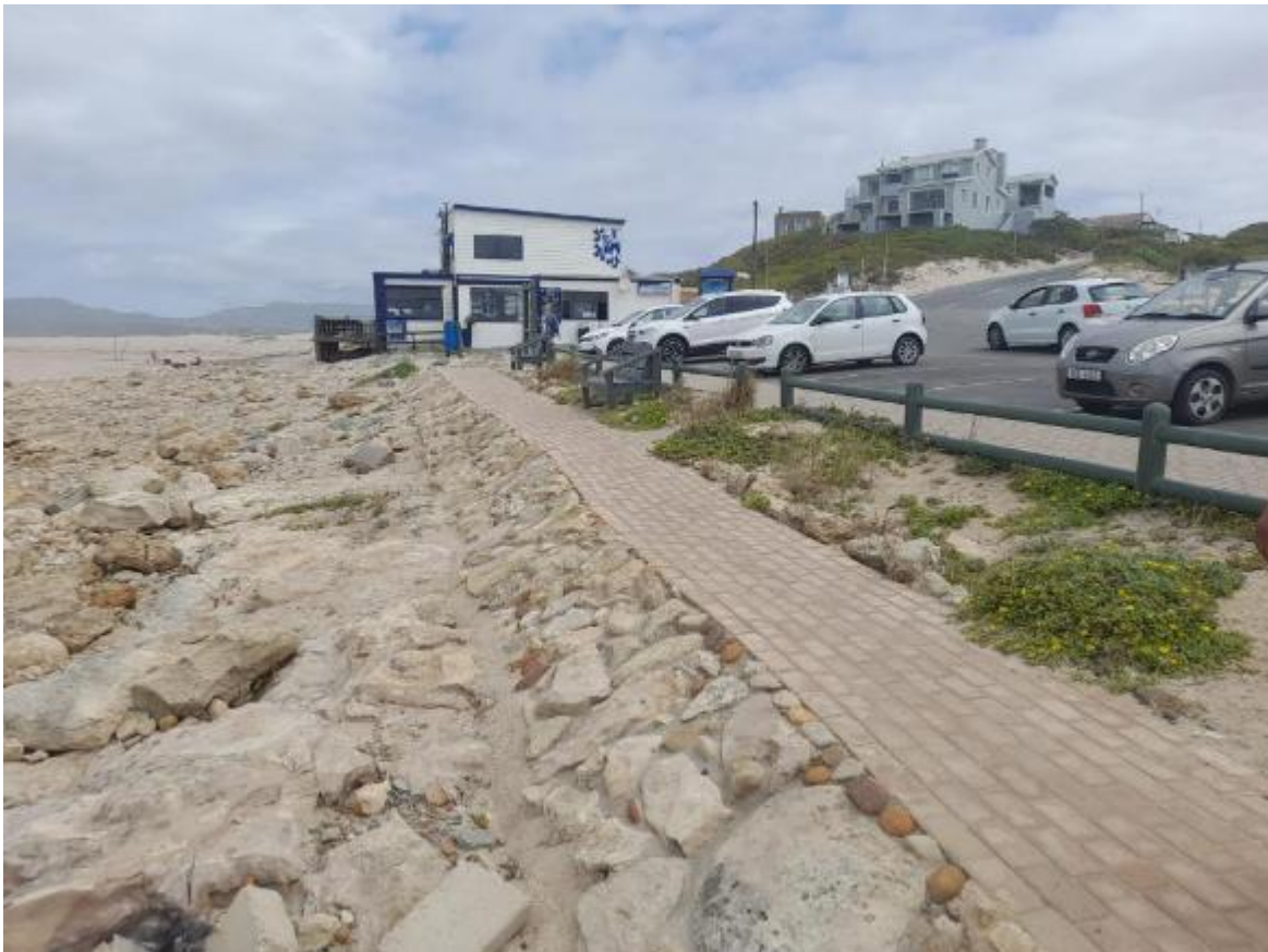
Figure 30 Paved walkway below parking area. Note sloped retaining 'seawall' on seaward side
