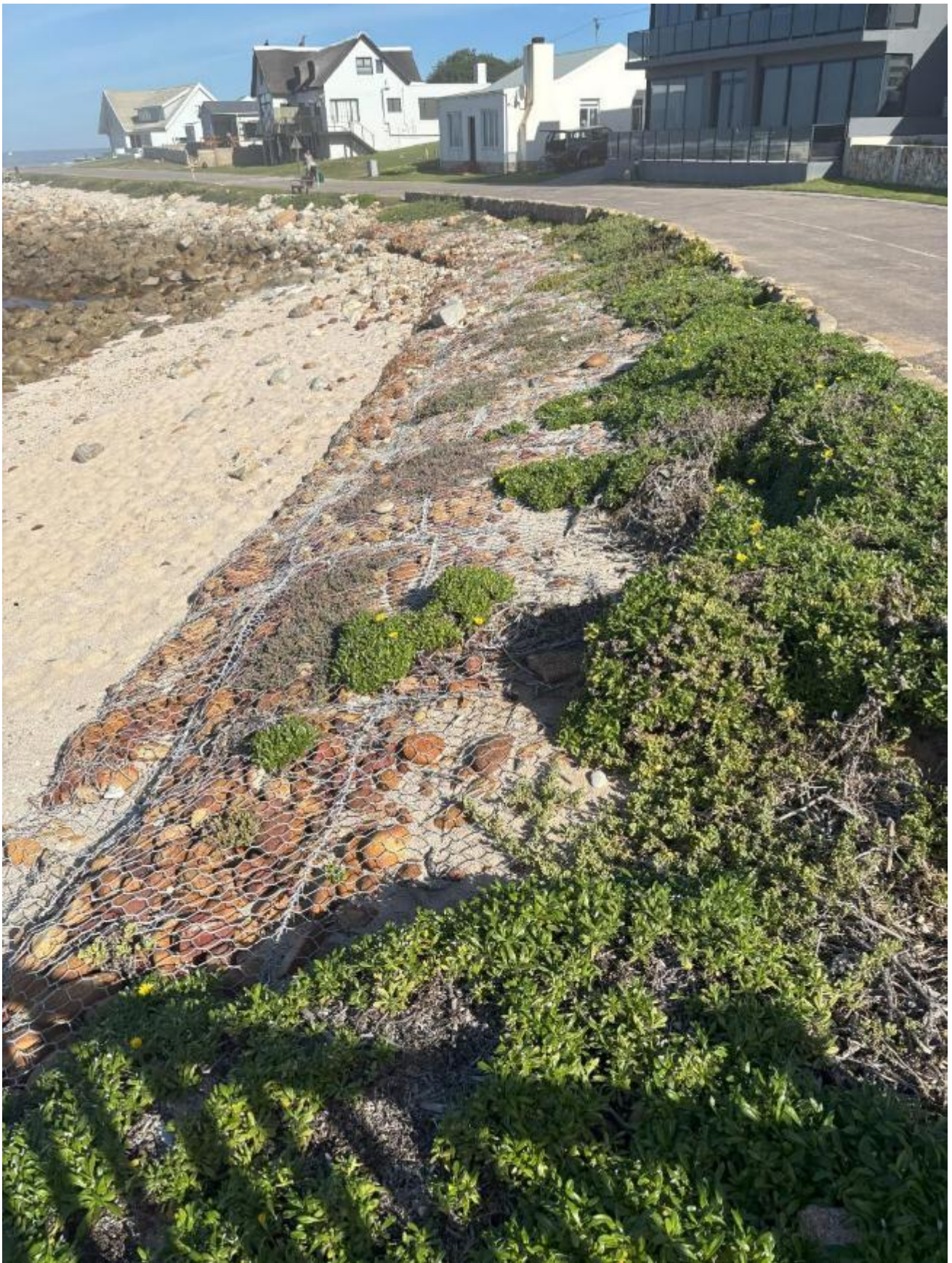
Figure 62 Southward view from access bridge at Ch570: Pedestrian-unfriendly gabion mattress verge above sandy beach area
