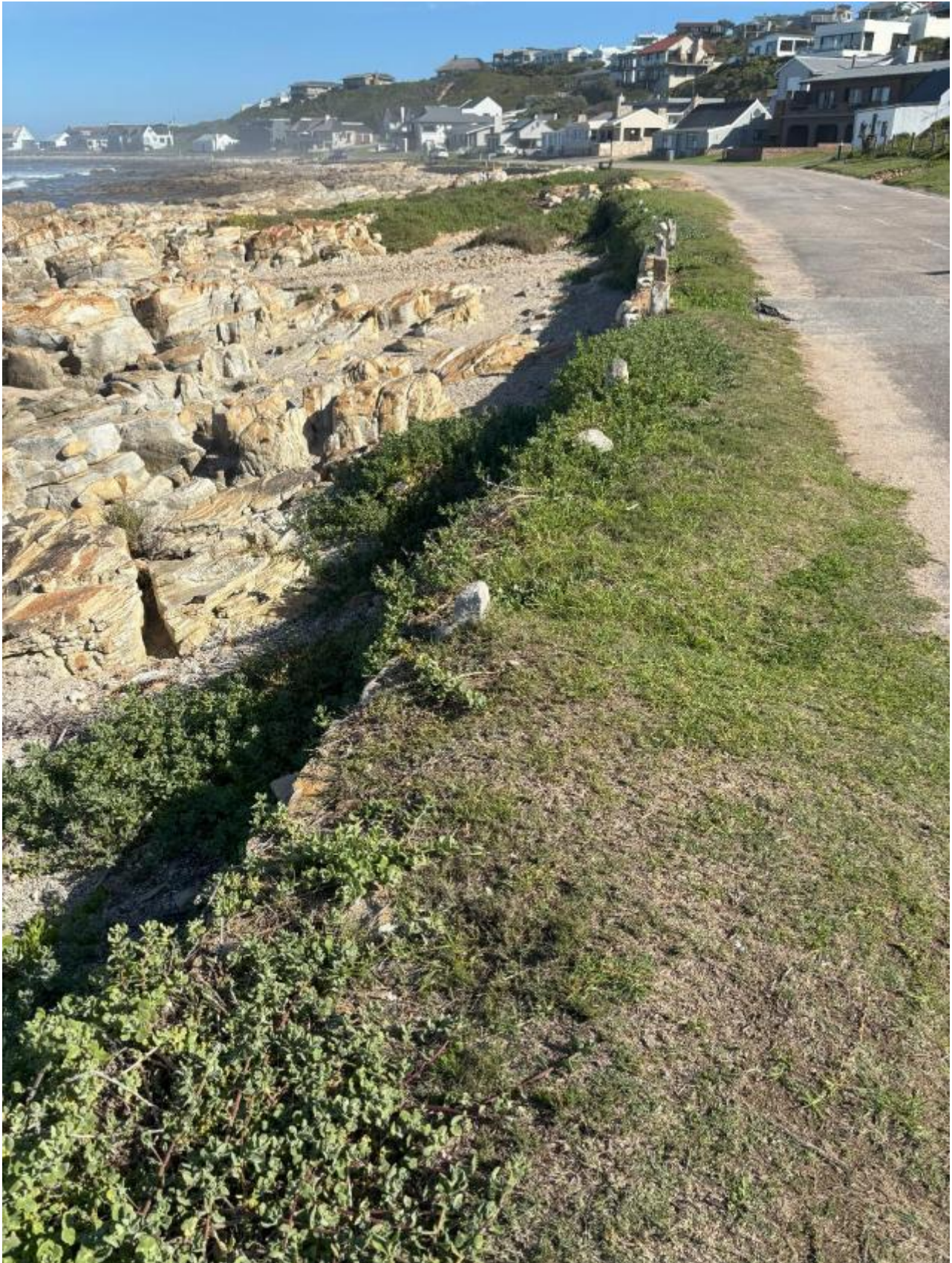
Figure 48 Southward view from Ch250: vegetated verge between 1.5 and 2m in width supported by natural rock masonry wall
