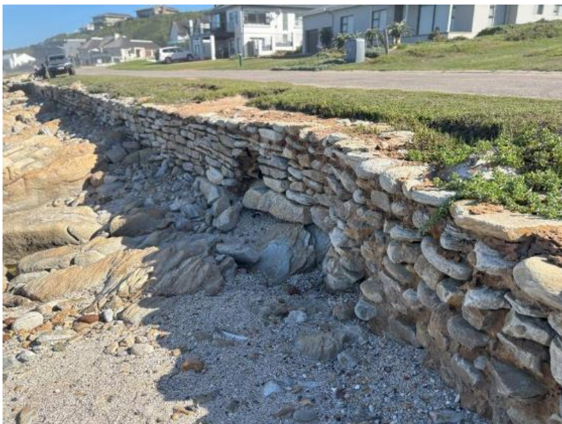
Figure 54 Vegetated roadway verge above natural rock masonry retaining wall around Ch450
