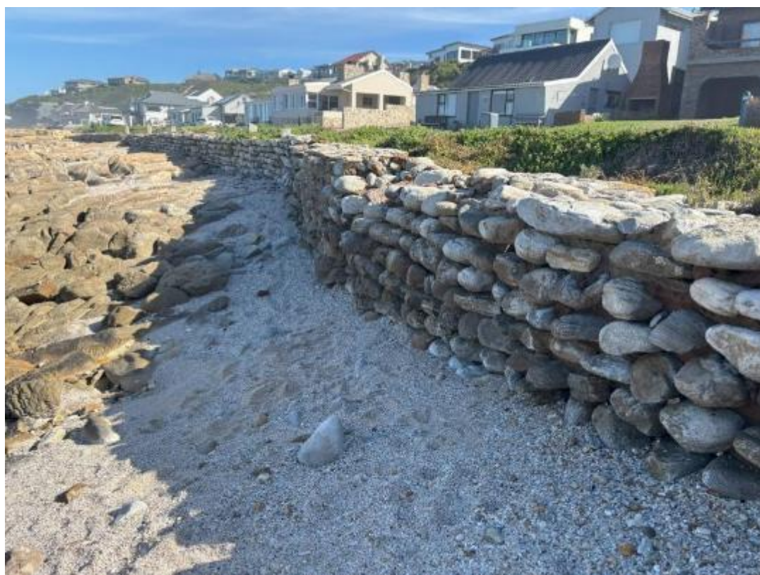
Figure 38 View from ocean side of natural rock masonry retaining wall from Ch320 southwards. Wall aesthetically pleasing and blends in with natural surroundings. Note however damage on top side from storm/flood events
