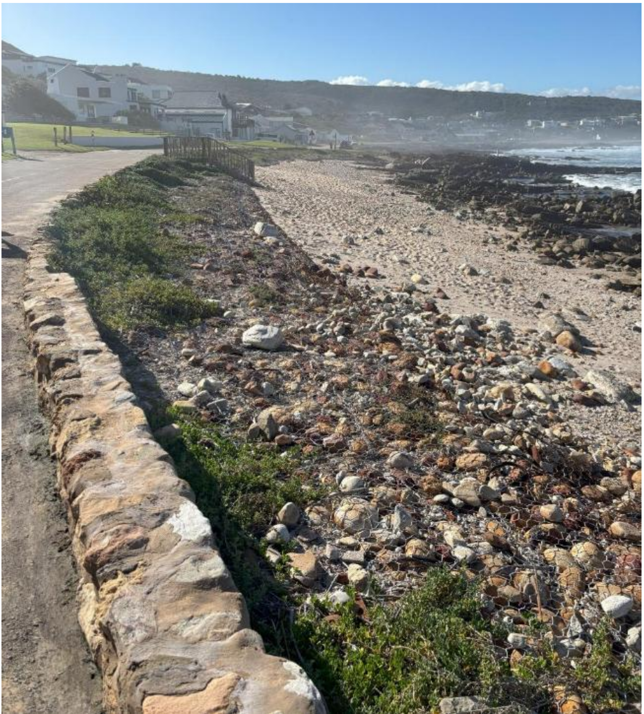
Figure 65 Northward view from Ch600: Note unsightly exposed and damaged wiring from gabion mattresses. Also newly reconstructed 'double' rock retaining wall in foreground This new wall has length of some 25m
