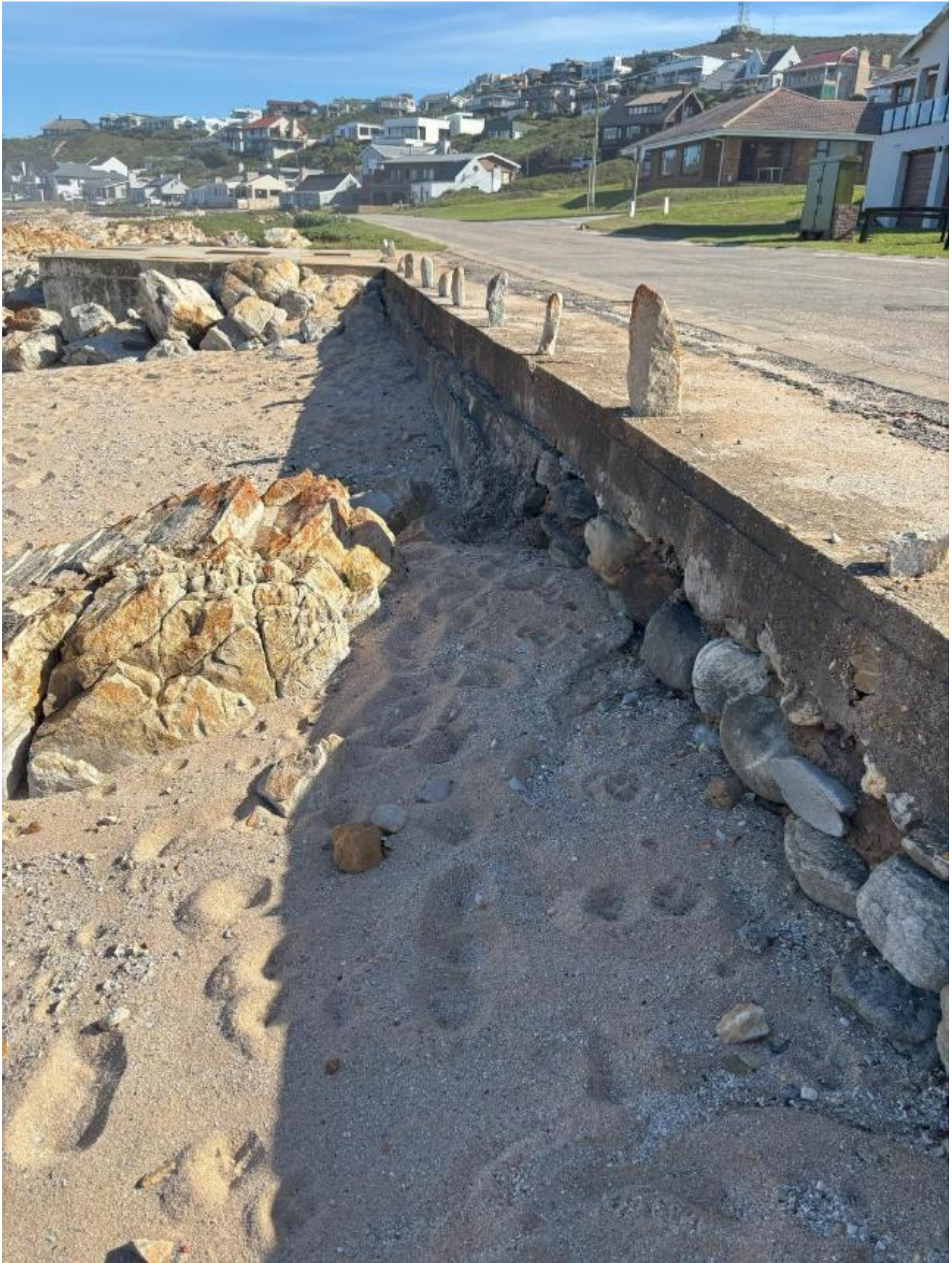
Figure 46 Southward view from Ch200. Note concrete encased sewerage pumpstation (?) and narrow concrete sidewalk/retaining structure with rock boulder foundation on sand(?). Innovative use of upright rocks in concrete as bollards
