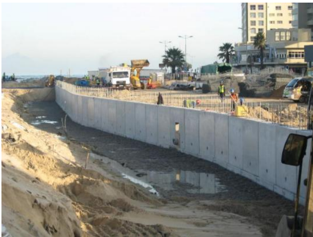
Figure 26 Seawall elements lined up. Seaward side. Note construction in the dry
