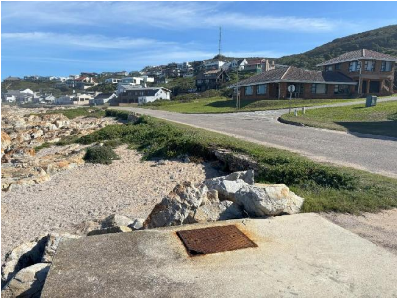
Figure 47 Southward view from pumpstation(?) slab approx. Ch210. Dolfyn Street intersection ahead. Large rock boulders as protection around pumpstation. Natural rock masonry wall adjacent to roadway
