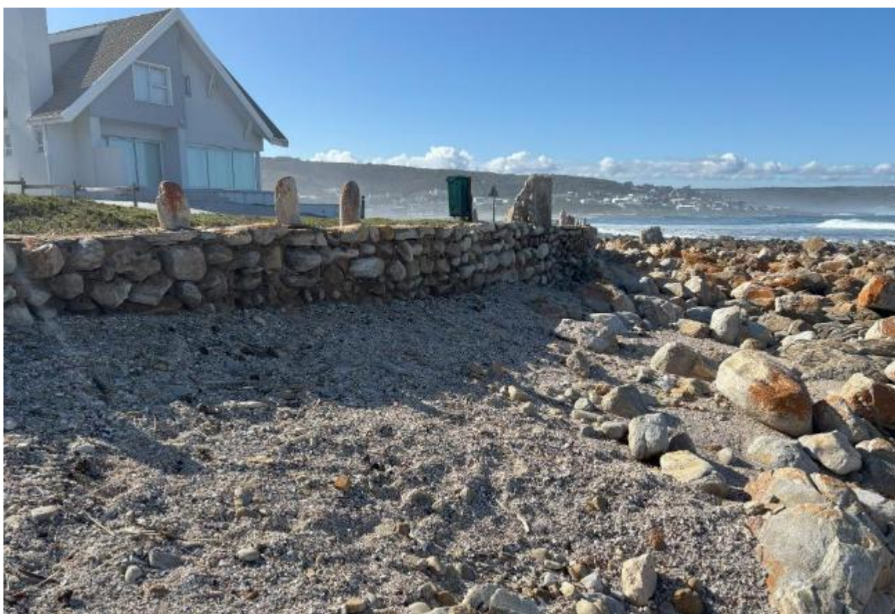
Figure 70 Natural rock retaining wall from seaward side at Ch780
