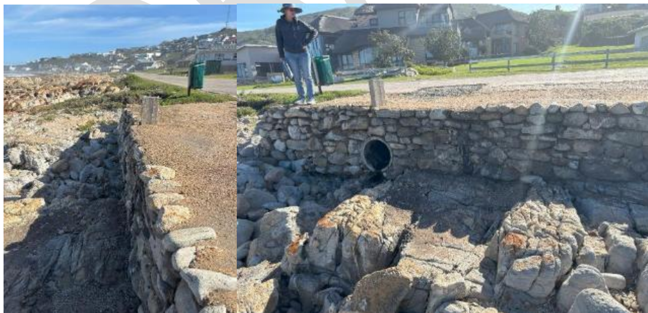
Figure 45 Concreted area with natural rock masonry retaining wall just past Ch150. Note storm water outfall
